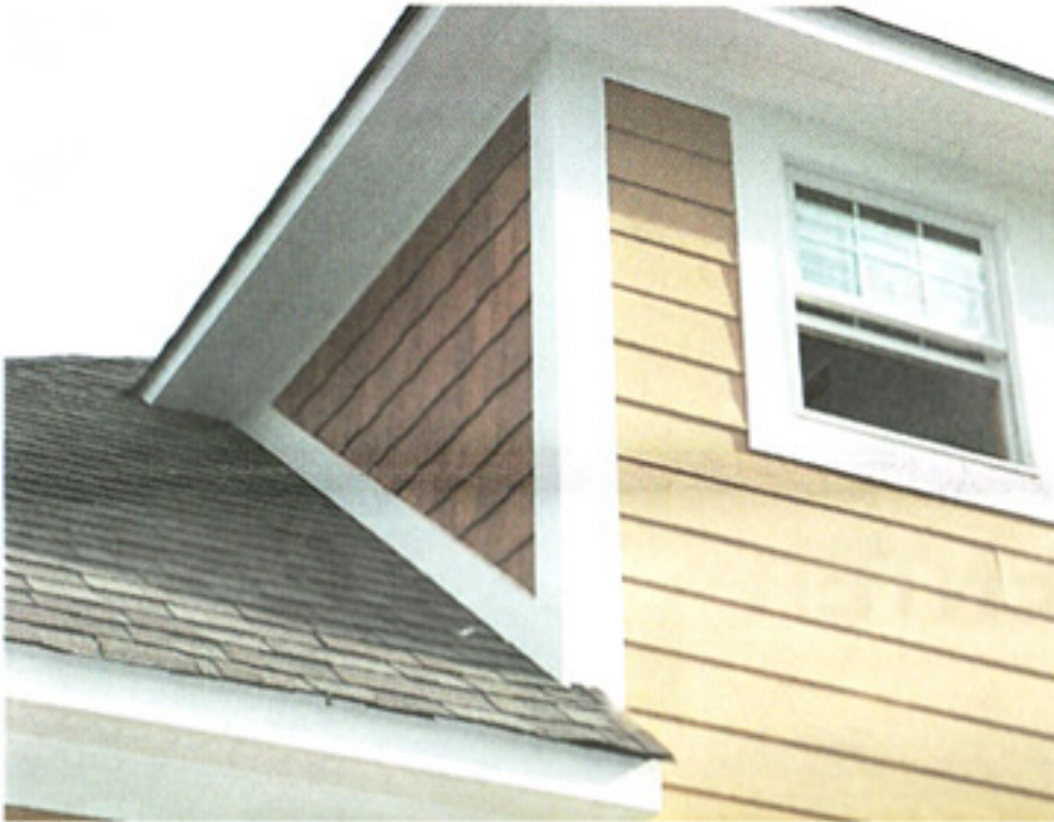
Certaainted Fiber Cement Siding™ makes a fiber cement siding made with a large portion of fly ash, a waste by product from coal.
