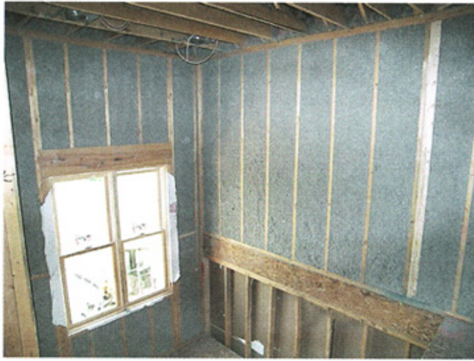
Cocoon™ Cellulose insulation is made with recycled paper, high in density and flame retardant. A blown-in cellulose insulation is environmentally responsible, can be less expensive and prevents the improper installation of fiber glass batts, leaving "cold pockets" in walls promoting condensation and possibly even mold.
