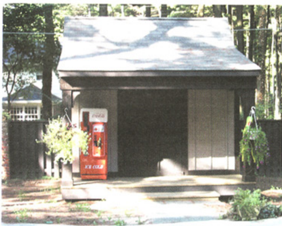
Storage area for pool equipment and misc. The owners first wanted to have a concrete foundation for the storage area. We then had a discussion and decided it would be best to do a cedar deck foundation for the storage area and how much better it would be for the environment. We are using more and more man-made materials for our projects. People are willing to pay a little more knowing that they are doing something good for the environment.
